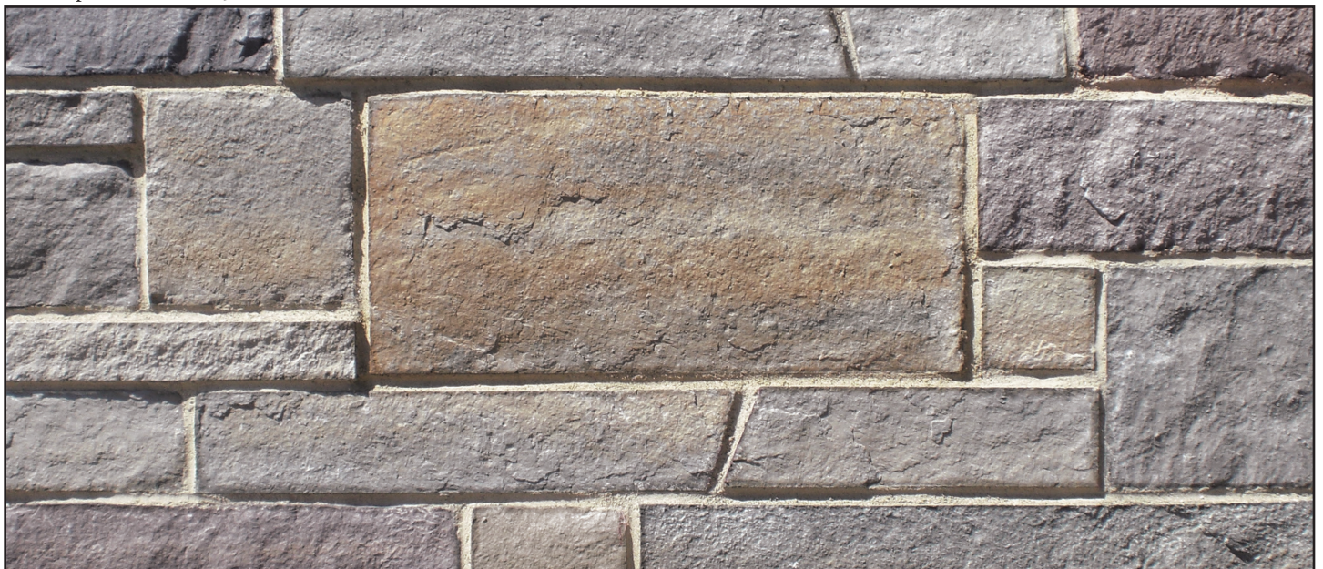
½" Deep Raked Grout Joint
